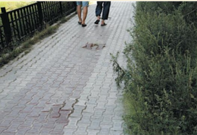
1.46 Ice heaving has damaged this pathway, made with pavers, in central Yakutsk, creating a hazard for pedestrians.
