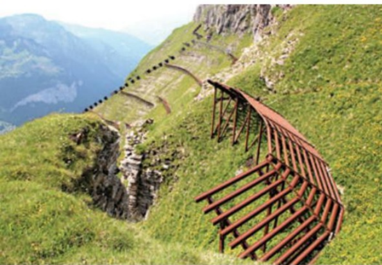
3.55 Fences on the slopes above the Lauterbrunnen Valley are designed to protect tourist settlements below from the hazards of snow avalanches.
