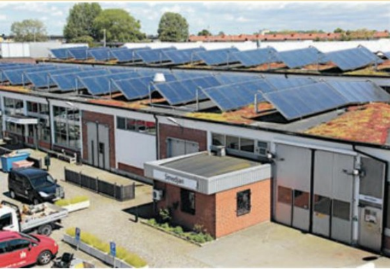
4.52 This factory in Malmö, Sweden, has a vast array of solar panels on its roof. Further insulation is provided with a green roof, which is a roof covered with vegetation planted over a waterproof membrane.
