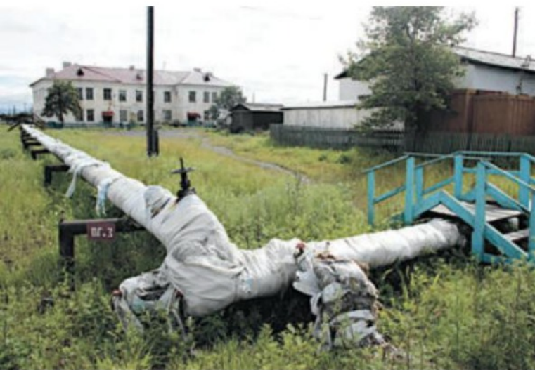
1.35 These water pipes in the Russian town of Artik have been built above the ground to avoid the inevitable breakage that would occur if they were buried in the permafrost. The pipes are insulated to protect them from the harsh weather, and a small bridge has been built so residents can use the pathway to get to their homes.
