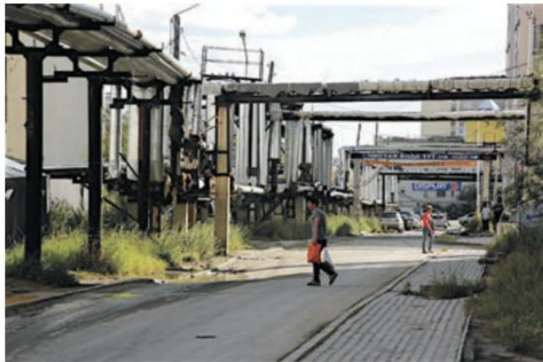
1.45 Buildings in Yakutsk are heated by hot water that is pumped in from a centrally located oil-fired boiler house. Overground pipes carry the hot water throughout the city, together with gas supplies and electricity lines, which form arches when they need to cross streets and roadways.
