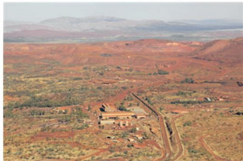
3.36 Mount Tom Price was the first iron ore mine to begin operations in the Pilbara after the iron ore export ban was lifted in 1960. The open-cut mine opened in 1966, and is operated today by Rio Tinto Iron Ore. Ore is extracted from the red hills in the middle of the photo and then processed on site before being transported by rail to the port of Dampier along the rail line in the foreground of the photo. It is a very capital intensive operation, and employs about 1,500 people to turn out its annual production of 28 million tonnes of iron ore.
