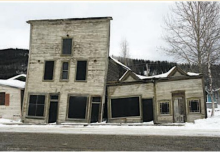
4.65 These buildings in Dawson City (Yukon, Canada) show what can happen when heated buildings are built on frozen permafrost. As a result of heating in the building, the permafrost melts, mixing soil with water, forming a paste into which the footings settle at different rates.
