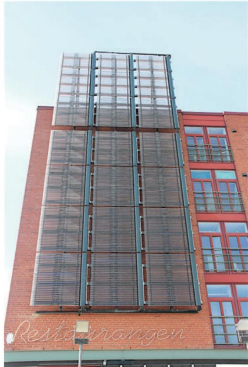
4.51 The side of this multi-storey building in Malmö, Sweden, is covered with evacuated solar hot water tubes. Compared with flat plate solar panels, evacuated solar tubes capture more sunlight because they have a greater surface area exposed to the sun. They can be used in sub-zero conditions and work in overcast conditions, making them suitable for cold environments.
