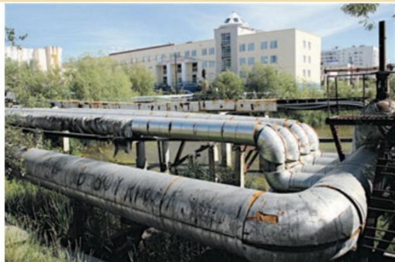
1.44 Large overground pipes near a housing estate in Yakutsk. The silver coating with the orange underlay is insulation.
