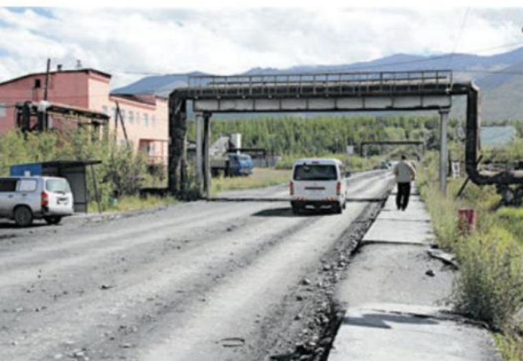
1.36 Service pipes have been built to cross over the main street of the small city of Ust-Nera in the Russian far east.
