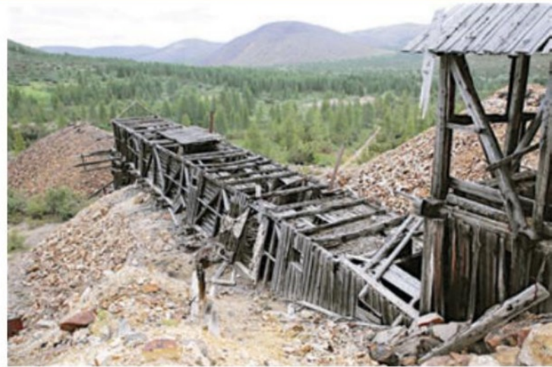
3.21 Another view of the abandoned Dneprovsky tin mine shows the large hills of tailings that have buried the natural landscape. Although the mine closed more than 60 years ago, the hills of mining waste remain devoid of any vegetation.
