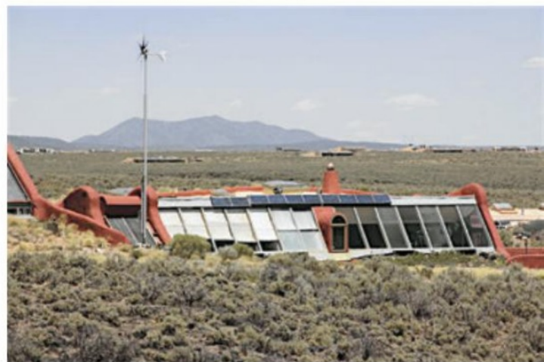
4.49 A typical house in the Earthship community near Taos, New Mexico, USA. The house has solar panels, a wind turbine and passive cross-ventilation.
