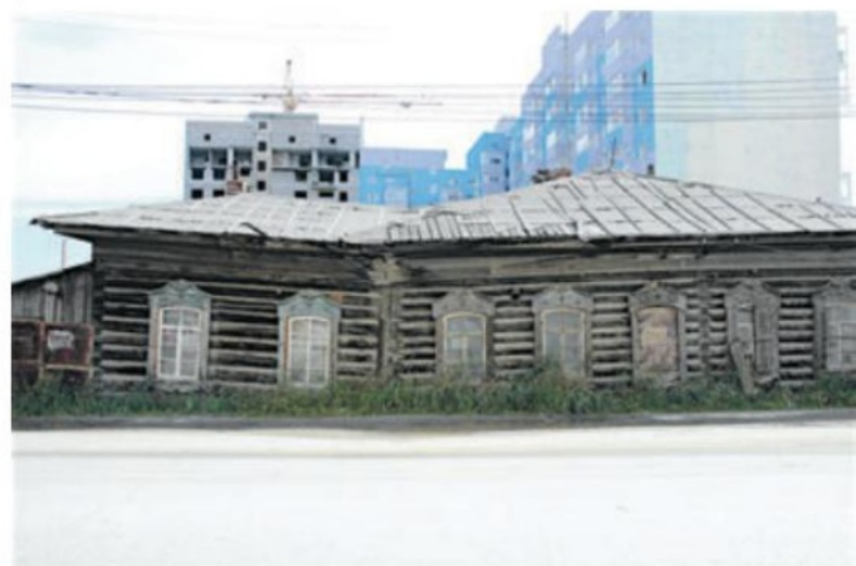
1.42 This old timber building in Yakutsk has suffered severe structural damage because of the unstable permafrost on which it was built. Examples of new high-rise concrete housing that are replacing the old timber buildings can be seen in the background.
