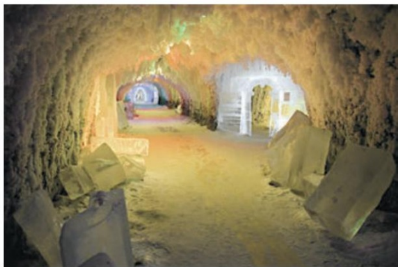
1.5 This tunnel beneath the Russian city of Yakutsk has been excavated through the permafrost. The build-up of ice on the tunnel walls is from the breath exhaled by people walking through the tunnel. The year-round temperature in the tunnel is a constant -8^{\circ}\text{C} , almost balmy in winter when the temperature outside may be -20^{\circ}\text{C} .
