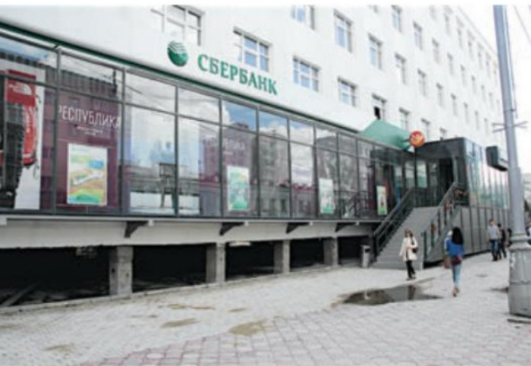
1.43 This new building, with shops and a bank on the lowest level and housing apartments above, shows the elevated construction used in Yakutsk to overcome some of the challenges posed by permafrost.
