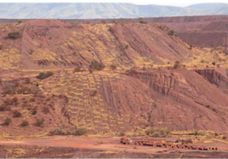
3.40 Stabilisation of steep slopes created during open-cut mining is needed to prevent erosion. Extensive erosion is evident on the side of this hill at Mount Whaleback, and native spinifex grasses are being planted in an effort to bind the loose soil to minimise further loss.
